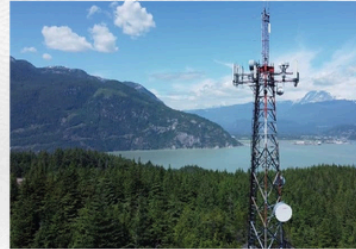
Telecom Base Station
